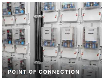
METERING AT SWITCHBOARDS
